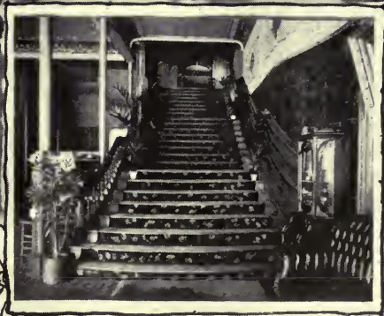
STAIRWAY OF KENYON
